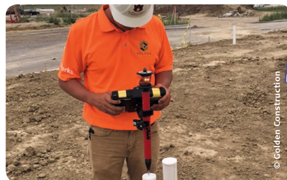
■ Laying out positions accurately with the Leica iCONstruct field solution.
