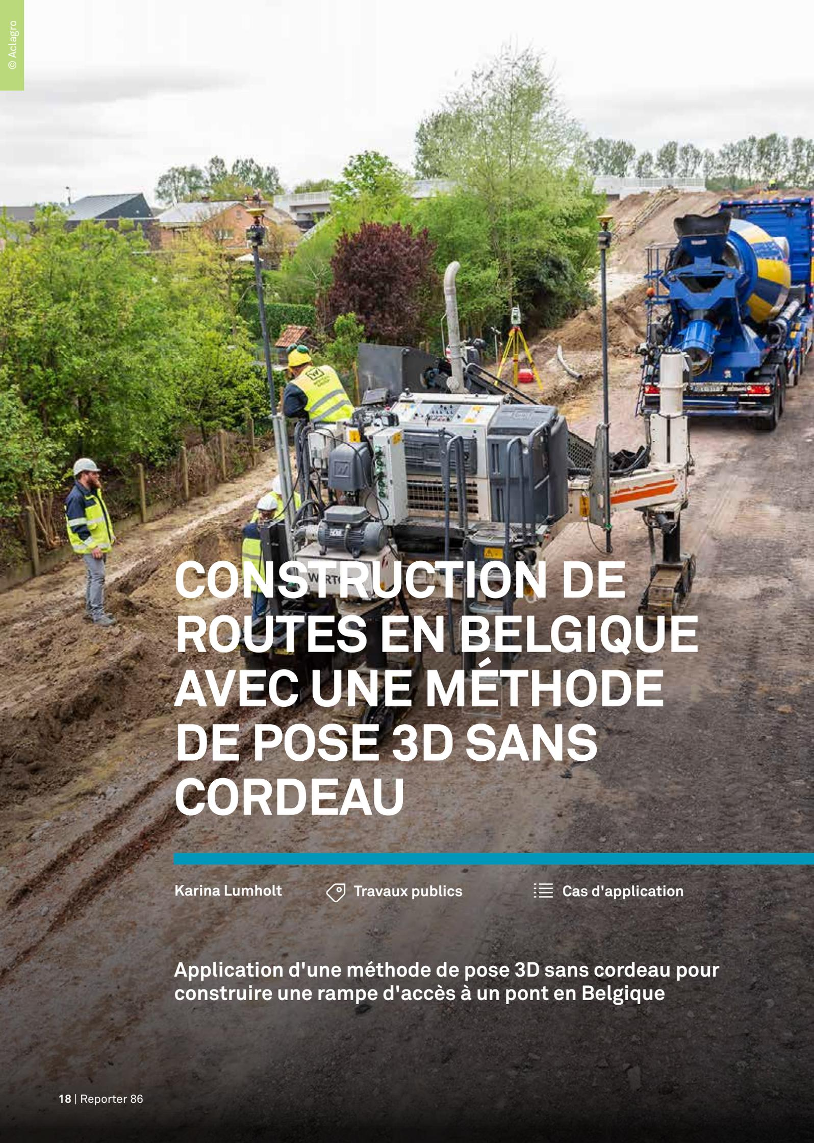
A construction site in Belgium showing a 3D paving machine (a large grey and white machine with a hopper) and a blue and yellow concrete mixer truck. Two workers in high-visibility vests and hard hats are visible. The machine is paving a concrete ramp. The background shows green trees and residential buildings under a cloudy sky.
