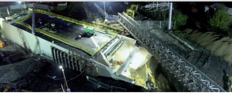
At 2 m per hour, the box tunnel is jacked into place.
