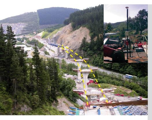
Arbizelay's bridge, 380 meters long, 6 spans high, 5 pylons and 12 meters wide is part of the AP-1 Vitoria - San Sebastián Motorway and is located near the city of Mondragon. Thanks to Leica GNSS technology, it was possible to successfully complete the manoeuvre of incremental launching of the bridge's deck over the pylons with an error of less than 3 centimetres.
