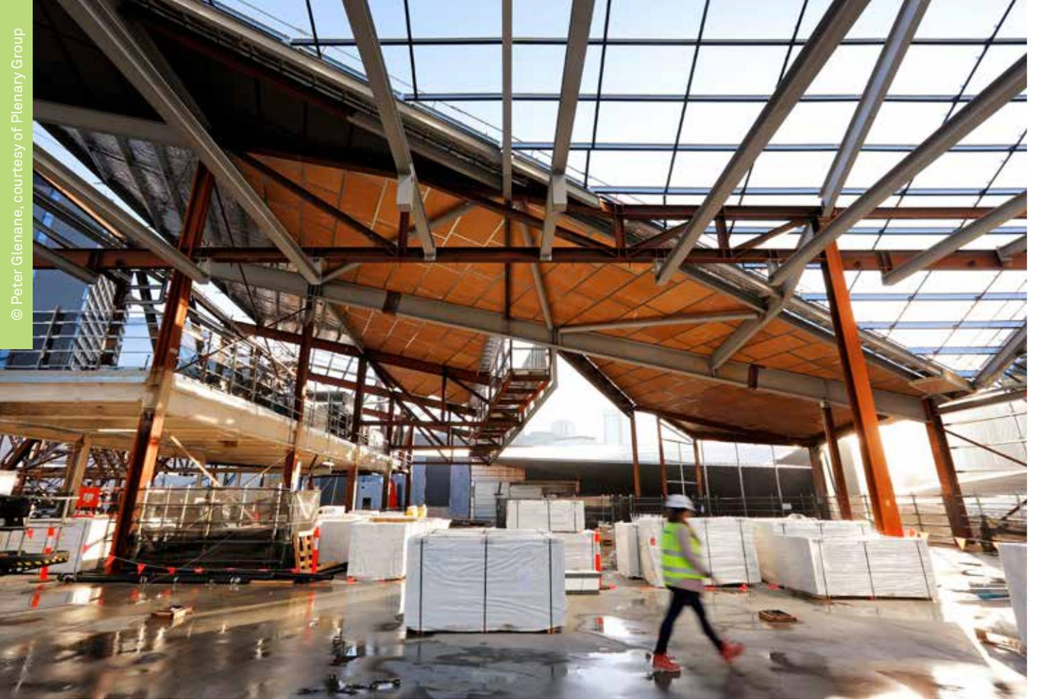
The method of steel erection proved to be a crucial time saving aspect allowing the façade contractor and concreter to proceed onsite unconstrained and work in parallel with the steelwork contractor. Stilcon site engineer Adam Tierney explained this ‘vertical method’ focuses on a full-height straight-up build of a section of the structure, which is replicated in turn across the building width adopting the same principal approach.
