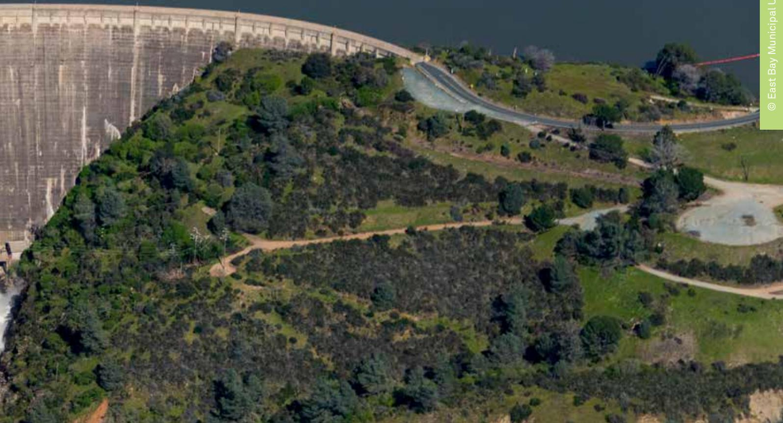
After a 4.4 magnitude earthquake in January 2018 on the Hayward fault centred in Berkeley, less than 8 km from the San Pablo dam site, EBMUD geotechnical engineers were able to log in to the AMTS automated monitoring system to **review whether there had been any actual movement or slumping on the dam**, and they confirmed that there was no significant movement. This ability to have information immediately and at their fingertips has proven to be a huge asset in managing dam safety at EBMUD.
